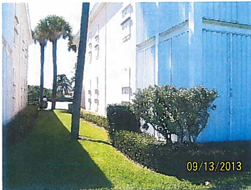
RIGHT SIDE VIEW (GARAGE DOOR OPENING)
