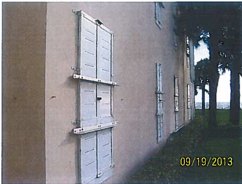
RIGHT SIDE VIEW (GARAGE DOOR OPENING)
