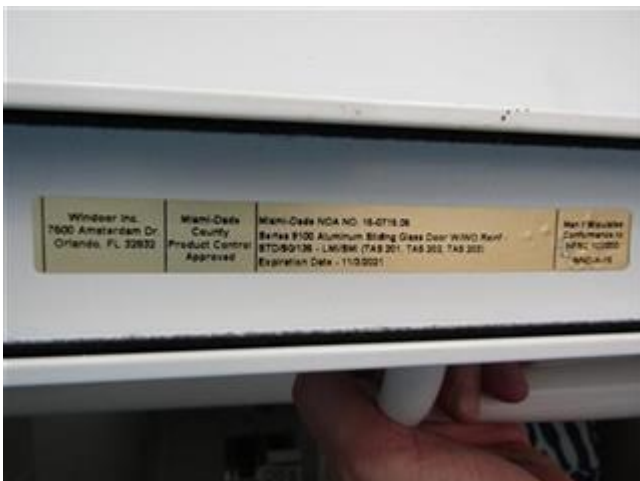
Hurricane Glass Doors Verification
