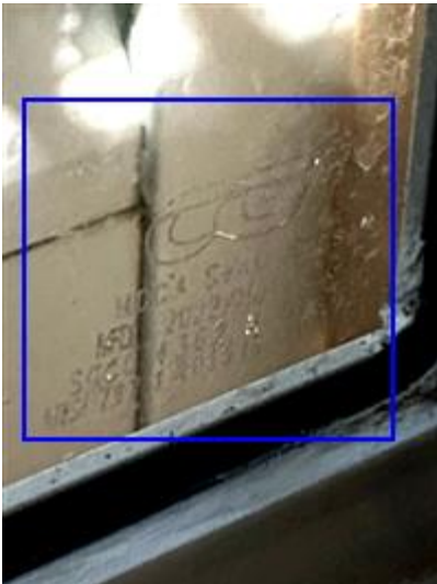
Hurricane Windows Verification
