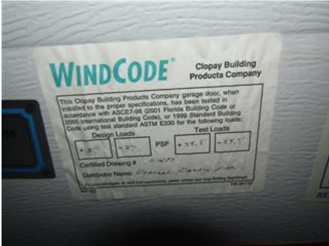
Hurricane Garage Door Verification
