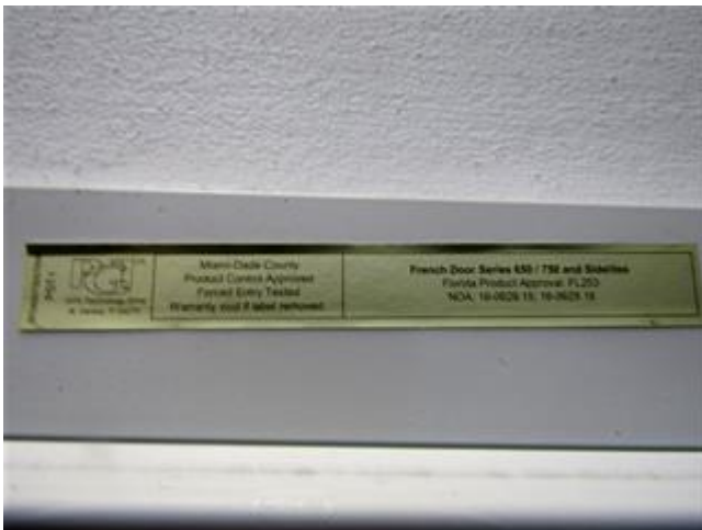
Hurricane Glass Doors Verification
