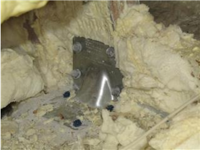
Roof to Wall Connection - Clips
