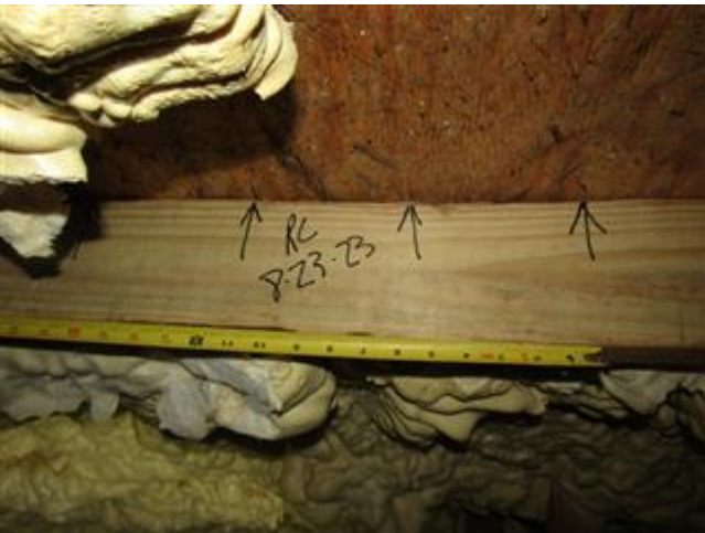
Roof to Deck Connection
