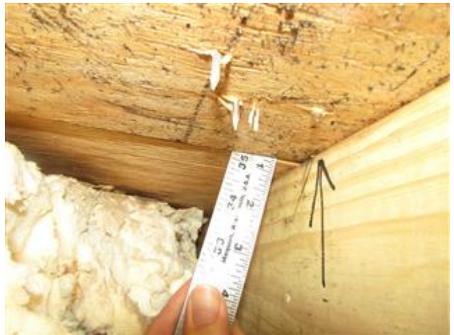
Roof to Deck Connection
