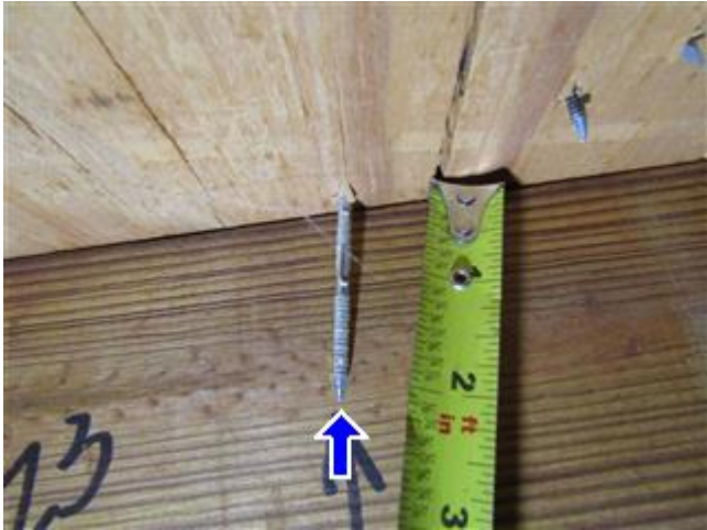
Roof to Deck Connection - 8D Nailing
