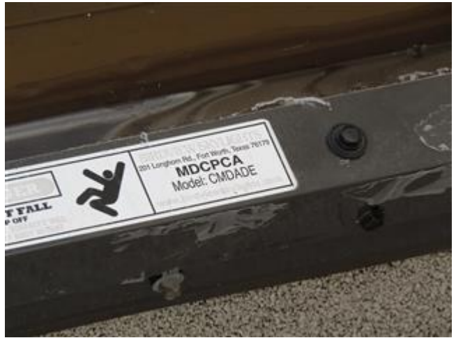
Hurricane Skylights Verification
