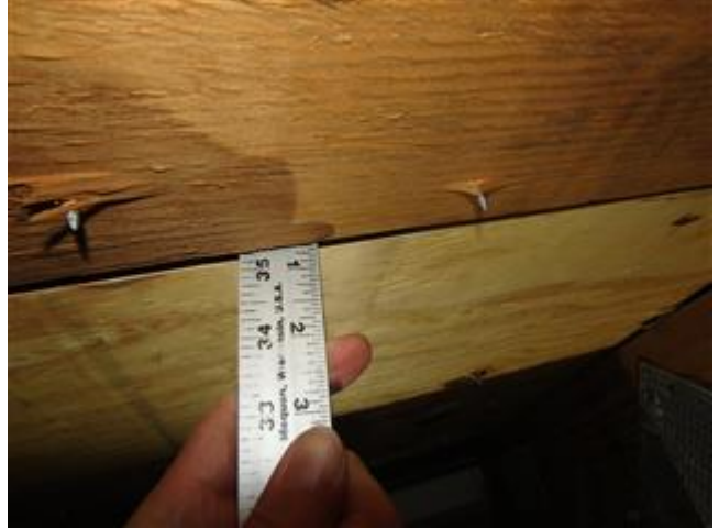
Roof to Deck Connection
