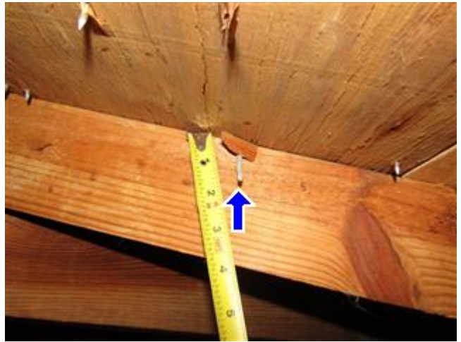
Roof to Deck Connection - 8D Nailing
