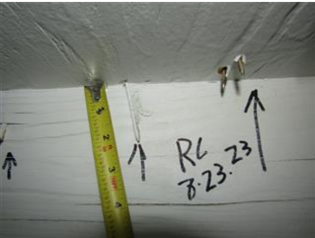
Roof to Deck Connection - 8D Nailing
