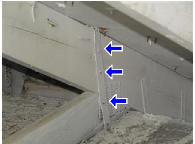
Roof to Wall Connection - Straps
