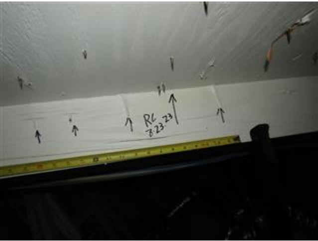
Roof to Deck Connection
