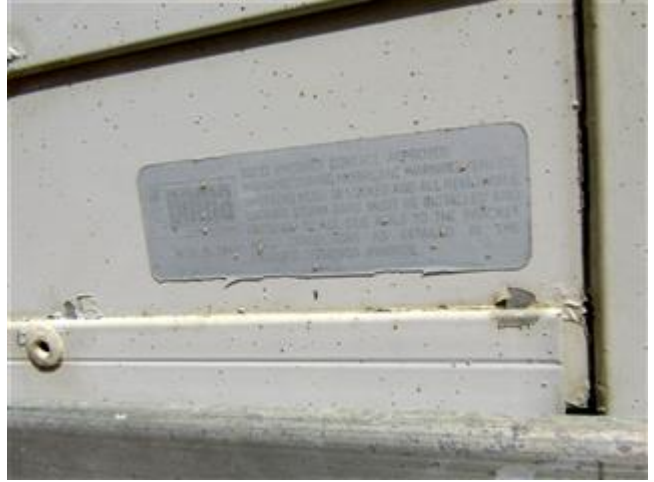
Hurricane Shutters Verification
