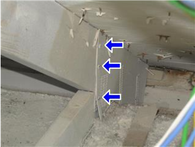
Roof to Wall Connection - Straps (Backside)
