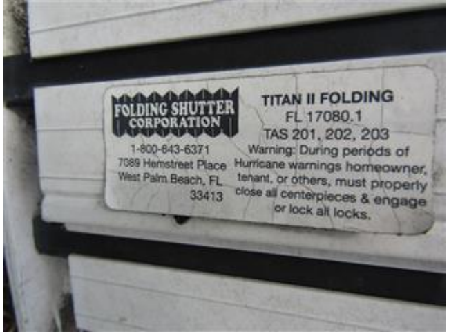
Hurricane Shutters Verification
