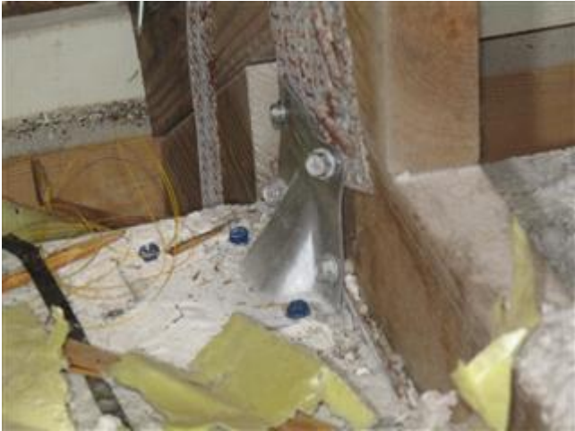
Roof to Wall Connection - Clips
