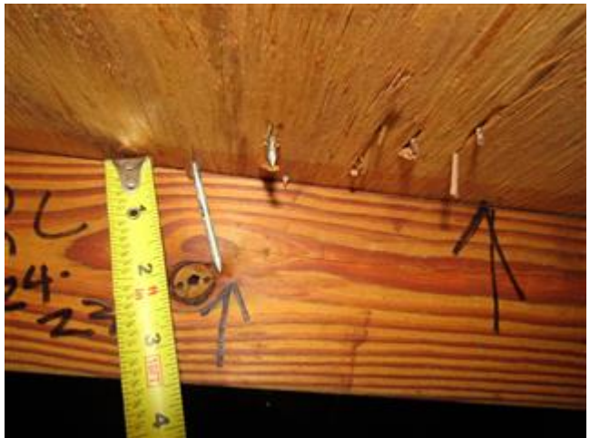
Roof to Deck Connection - 8D Nailing
