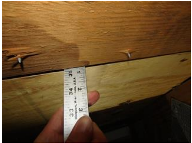
Roof to Deck Connection
