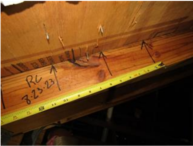
Roof to Deck Connection
