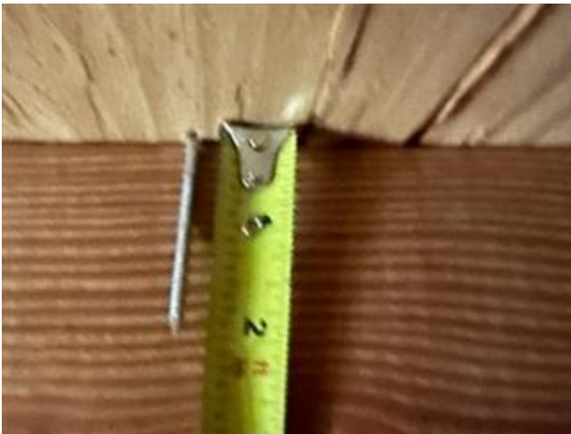
Roof to Deck Connection - 8D Nailing
