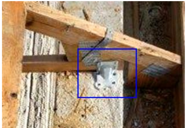
Roof to Wall Connection - Clips
