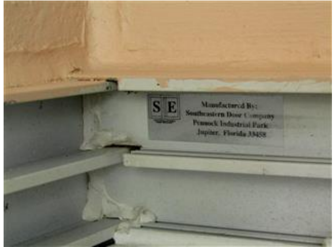
Hurricane Shutters Verification
