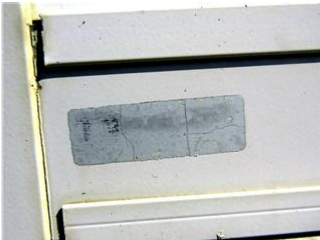
Hurricane Shutters Verification
