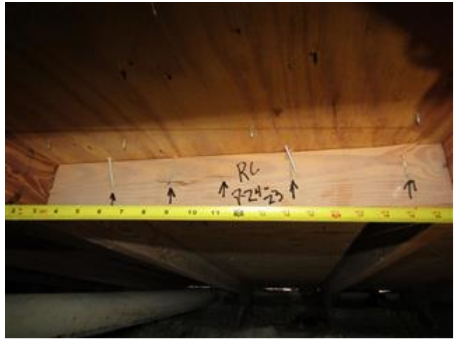
Roof to Deck Connection
