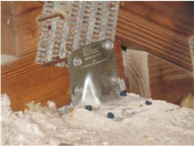
Roof to Wall Connection - Clips
