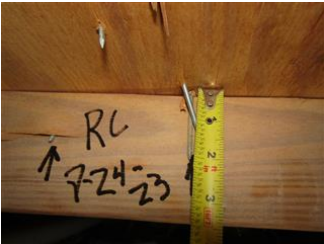
Roof to Deck Connection - 8D Nailing
