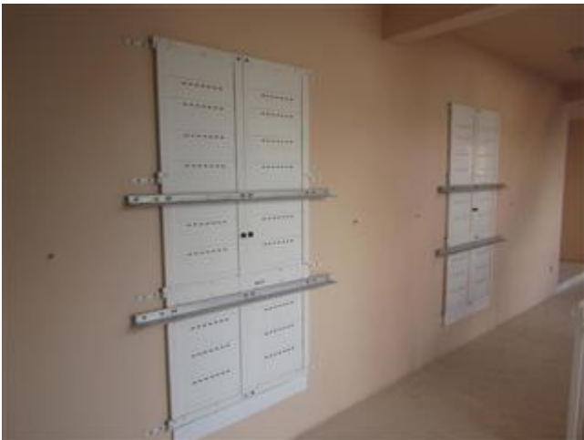
Hurricane Shutters Windows
