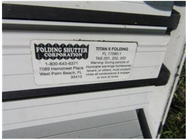
Hurricane Shutters Verification
