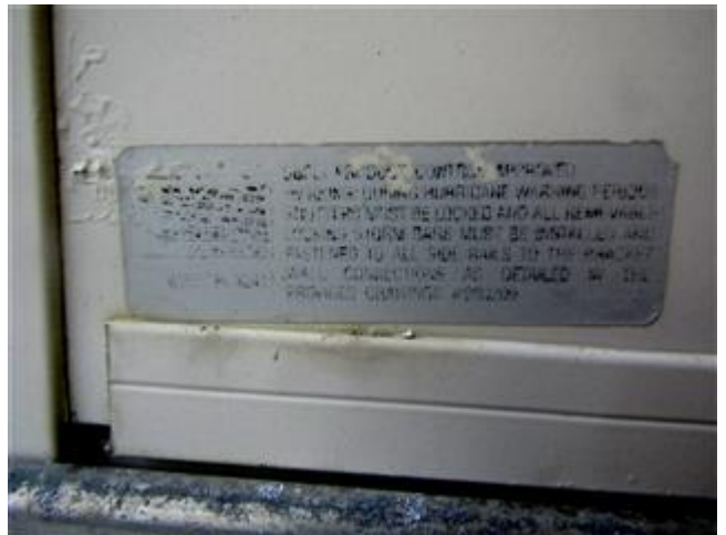
Hurricane Shutters Verification
