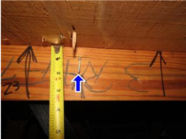
Roof to Deck Connection - 8D Nailing
