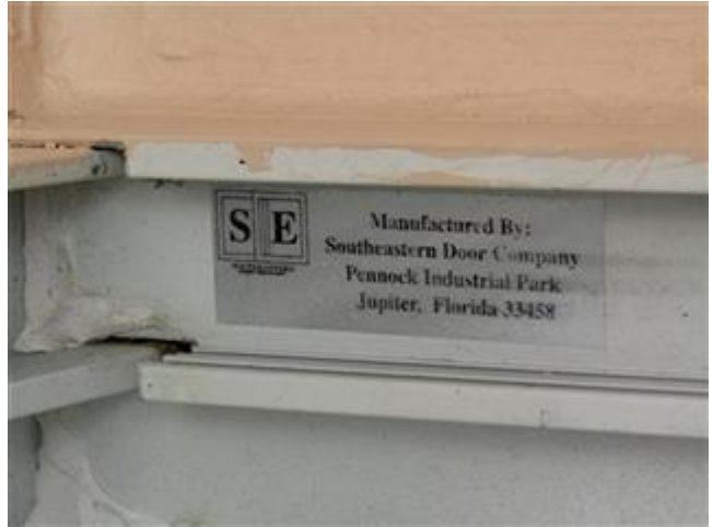
Hurricane Shutters Verification
