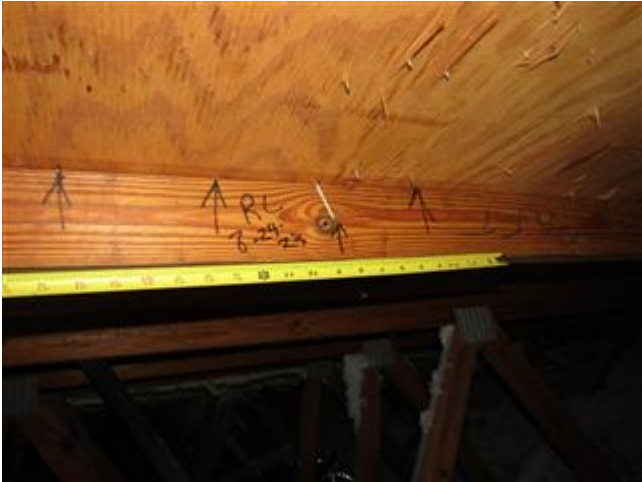
Roof to Deck Connection
