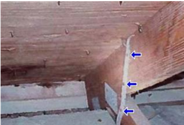
Roof to Wall Connection - Straps
