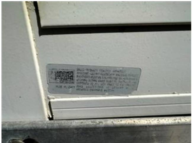
Hurricane Shutters Verification
