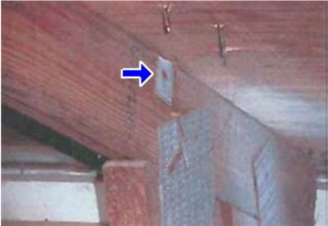
Roof to Wall Connection - Straps (Backside)
